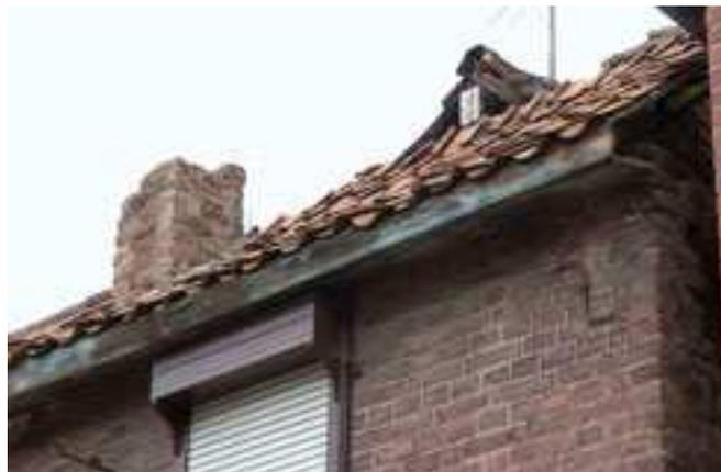
Figure 6.3: Slight damage onto buildings (broken chimneys and damaged roofs) could be observed in the epicentral region of the  $M_L$  4.9 2002 Alsdorf earthquake (after Hinzen (2002)).
