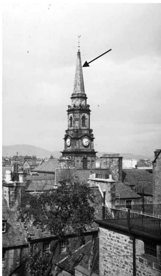
Figure 2. The spire of Inverness Jail. This picture was taken after the spire was restored. Arrow indicates approximately where the rotation occurred “within 5 or 6 feet of the top, the angles of the octagon turned nearly to the middle of the flat sides of the octagons underneath it” (Anonymous, 1816). This photograph is available as part of the Highland Photographic Archive (see Data and Resources section). Sense of rotation unknown.
