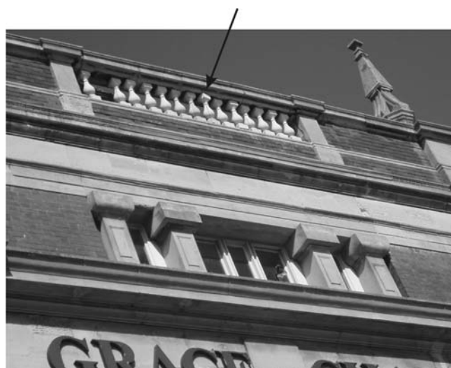
Figure 7. Balustrade support at Grace Chapel, Folkestone, rotated counterclockwise out of position (Sargeant, NERC, 2007).
